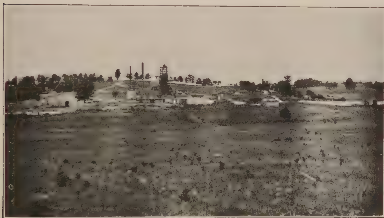
(18) Modern mine plant and company cottages at Franklin mine.
